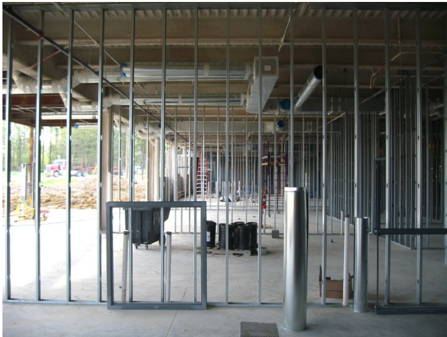
First, Second, Third Floor (Column Lines 1-5) Metal Stud Walls are Ongoing.
