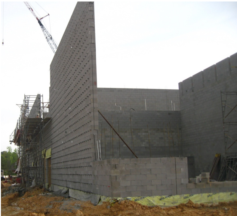
Full Height CMU Walls throughout the South West Building Are Ongoing
