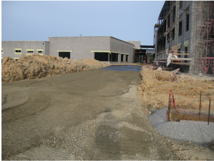
Installation of Access Roads Ongoing
