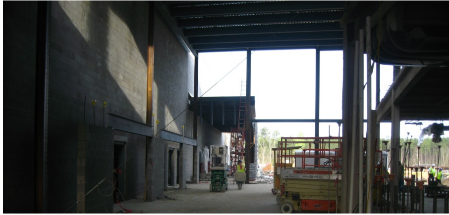
Installation of Structural Steel (South Building Column Line G) is Ongoing
