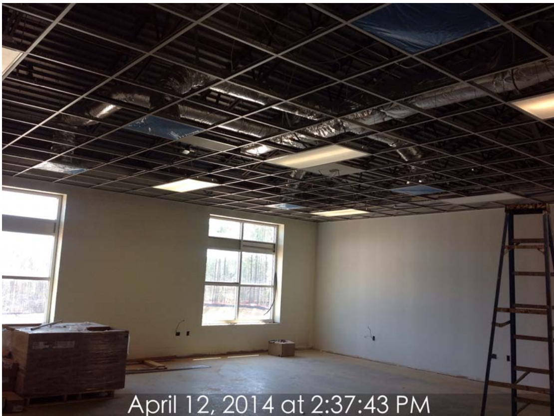
Figure 9: Area 2200 MEP to ceiling grid finishing for next week's inspection
