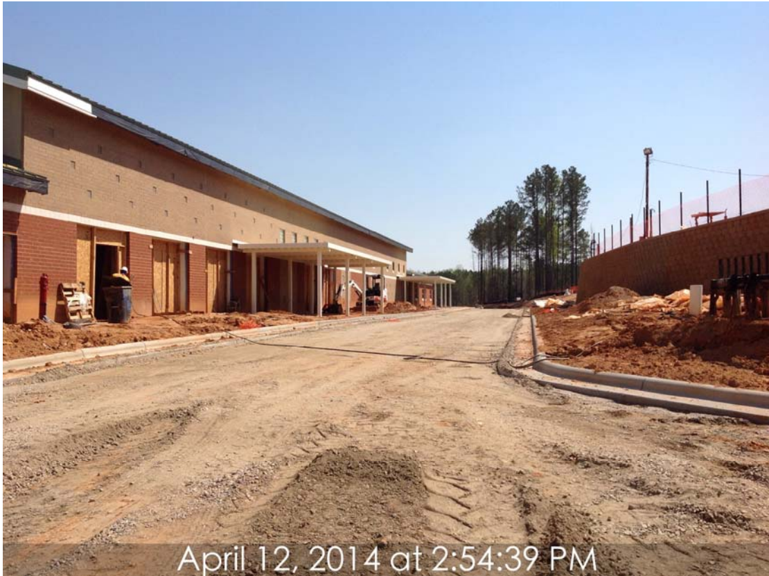
Figure 2: Area 100 West at Bus loop stone base set up for paving
