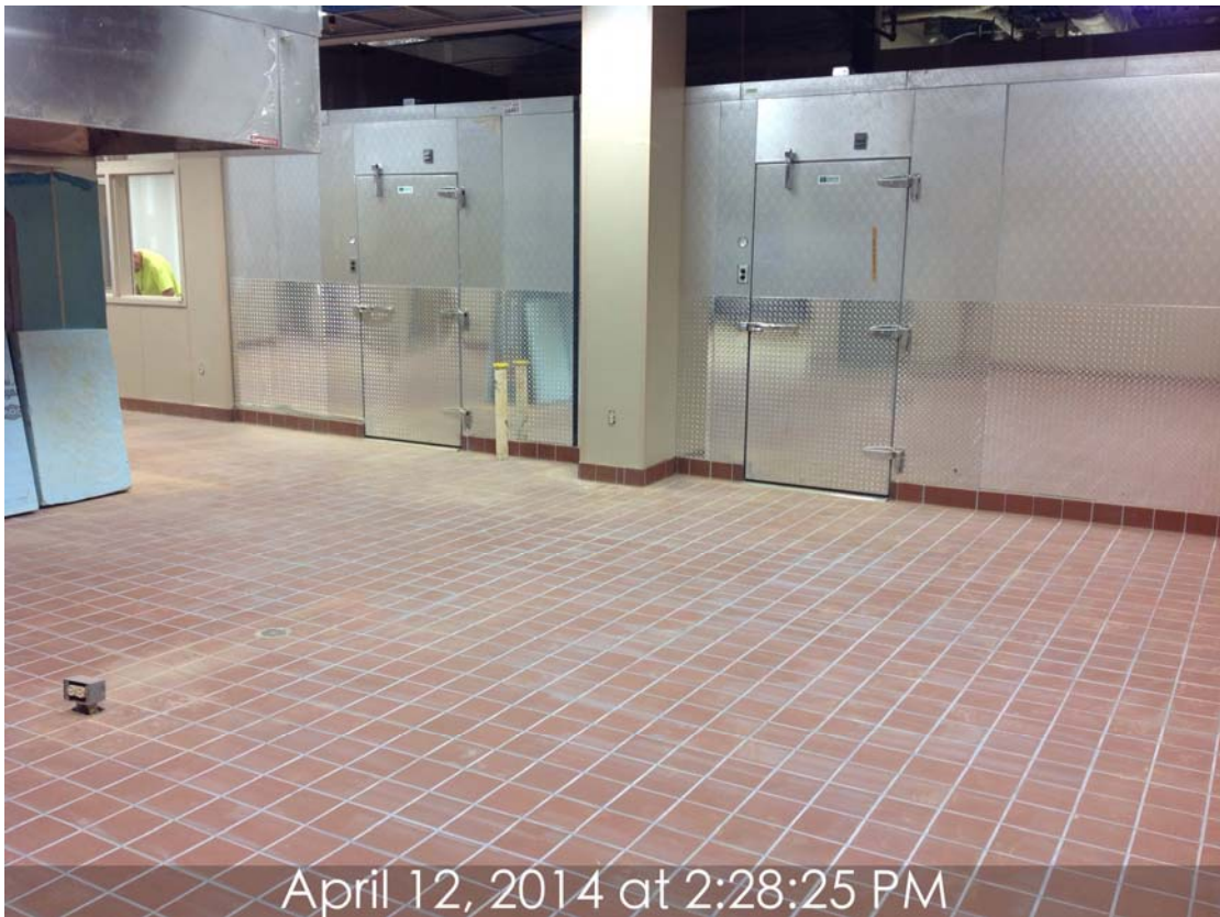
Figure 6: Area 100 Kitchen being cleaned in preparations for equipment delivery
