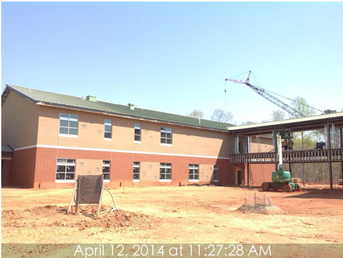
Figure 4: Area 200-300 connector finishing stud framing for mason next week
