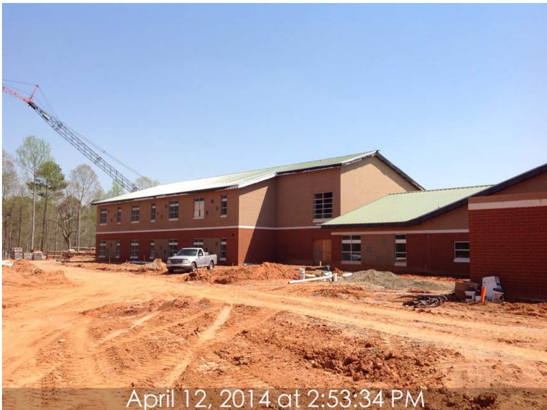
Figure 3: Area 300 North finishing grading of fire lane
