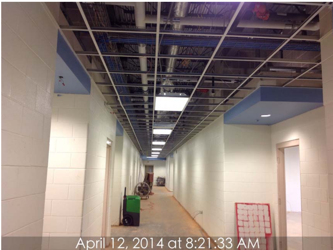
Figure 7: Area 200 main corridor, preparing for overhead inspections next week
