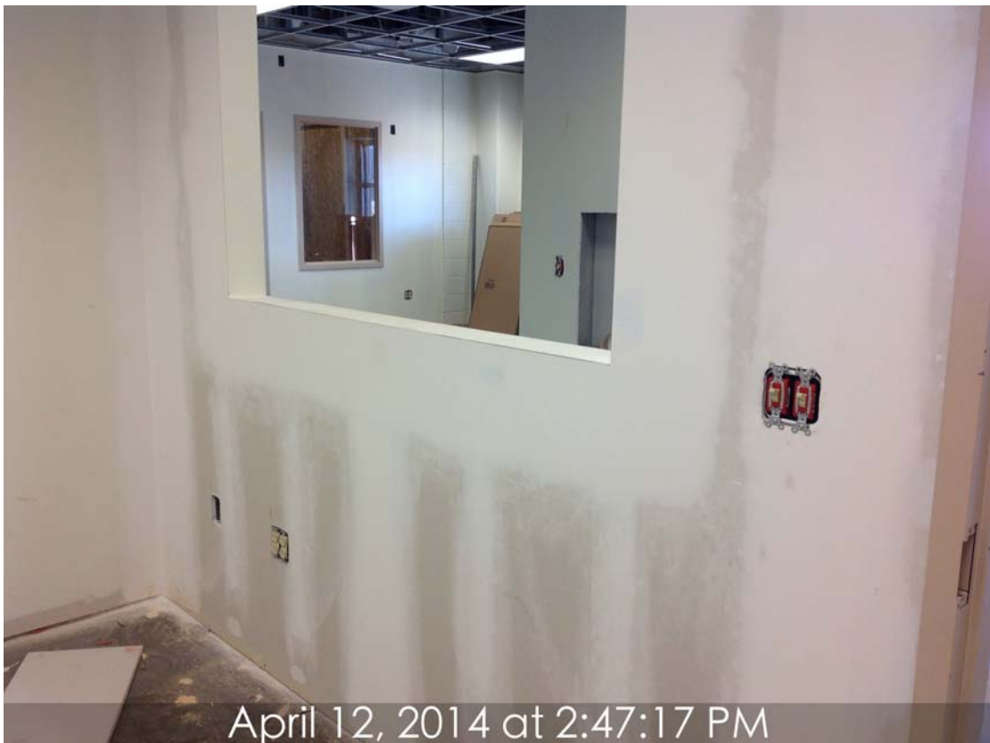
Figure 5: Area 100 Drywall finished for paint and electrical trim out started
